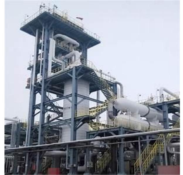
The reactor used for methanol synthesis is the most crucial part of the process, as it is not only responsible for the reaction itself, but also for removal of heat generated during the process . Current reactor designs for methanol synthesis are mostly fixed-bed gas phase technologies, which can be either characterized thermodynamically, by cooling type, or by flow design . Fluidized-bed gas phase, liquid phase and membrane based technologies are emerging
